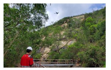
At Pillar Point Valley Restorated Landfill in Hong Kong, regular inspections of slopes and surface channels are required. This involves high-level climbing and photography, posing risks of heat stroke and working at height. In 2024, we introduced drones for inspections, eliminating these risks and saving 2-3 days of inspection time, significantly improving safety.
